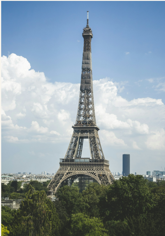
Eiffel Tower in daylight. Photograph: Guillaume Bleyer / Unsplash.
